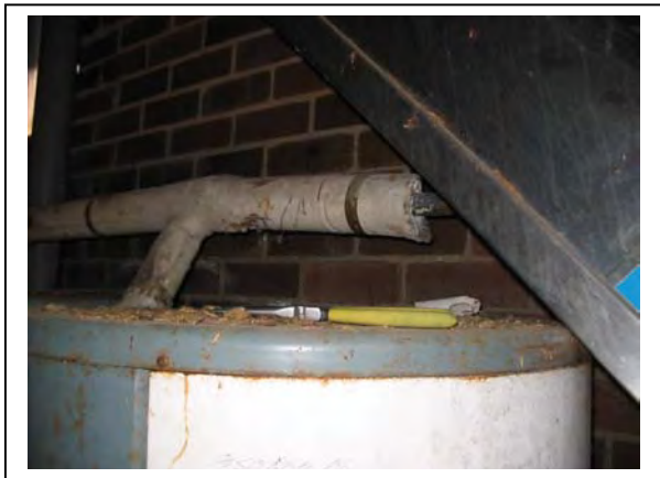
Plates 3 & 4: Pipe Lagging to Hot Water Pipes in Cafeteria Plant Room
