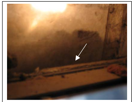
Plate 6: Asbestos cement sheet - Block 2 3 rd Floor sheet behind lift indicator panel.
