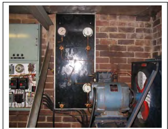
Plate 8: Asbestos Electrical Board - Cafeteria Air Handling Unit Plant Room.
