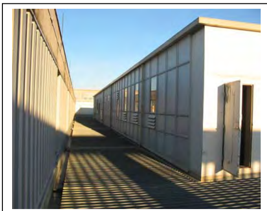
Plates 7: Asbestos Cement Sheet – Block 2 Exterior Plant Room.
