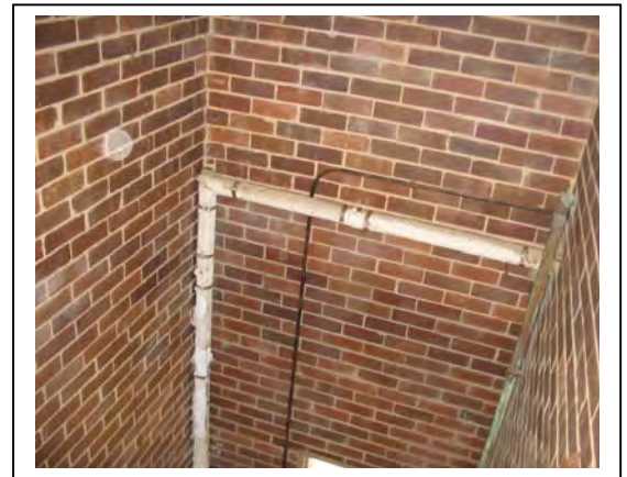
Plates 3 & 4: Pipe Lagging to Hot Water Pipes in Cafeteria Plant Room
