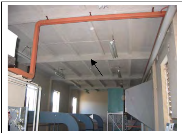
Plates 1 and 2 : Plant Room limpet spray insulation on ceiling and wall pillars
