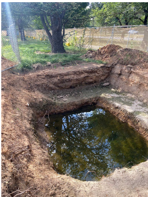
Excavation within TPZ. A review of the roots cut during this dig showed a minimal amount of roots above 20mm diameter were cut.
