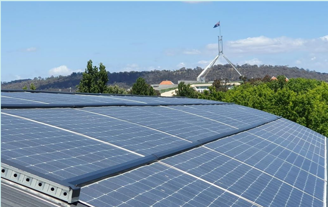
Figure 1: Polycarbonate solar panels on Questacon's curved roof
